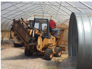
Installing the Fish Pond
